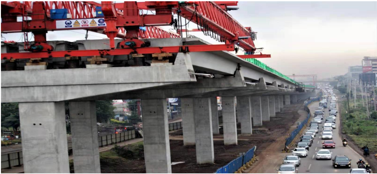
An express highway under construction
